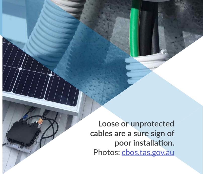
Loose or unprotected cables are a sure sign of poor installation.
